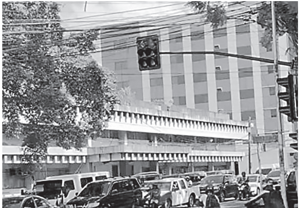
NEW TRAFFIC LIGHT. The new traffic signal lights along the North Capitol Road in Bacolod City during its test operation in the first week of January 2024. Traffic lights equipped with radar sensor technology are to be fully operational in the initial three main intersections of the city this week. (Contributed photo)
