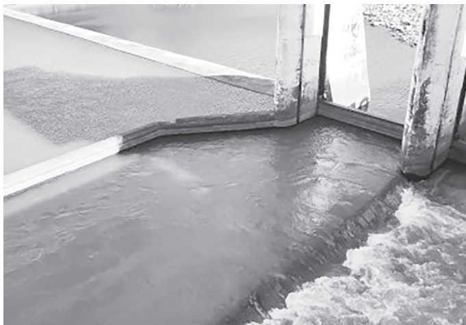
IRRIGATION DAM. A portion of the Bago River Dam, which supplies water to the Bago River Irrigation System (BRIS) in Negros Occidental, in this photo taken end of February. The BRIS serves six local government units with a total program area of 10,920 hectares. (Photo courtesy of NIA-Negros Occidental Irrigation Management Office)
