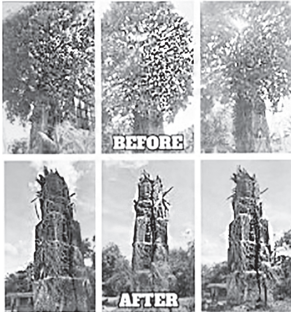
RESTORED. Before and after photos of the historic “simboryo” or smokestack of a muscovado sugar mill in Barangay VIII, Victorias City, Negros Occidental. Previously, the structure was “engulfed by overgrown vegetation that obscured its architectural beauty and historical value”, the city government said on Monday (March 11, 2024). (Photo courtesy of Councilor Dino Acuña)
