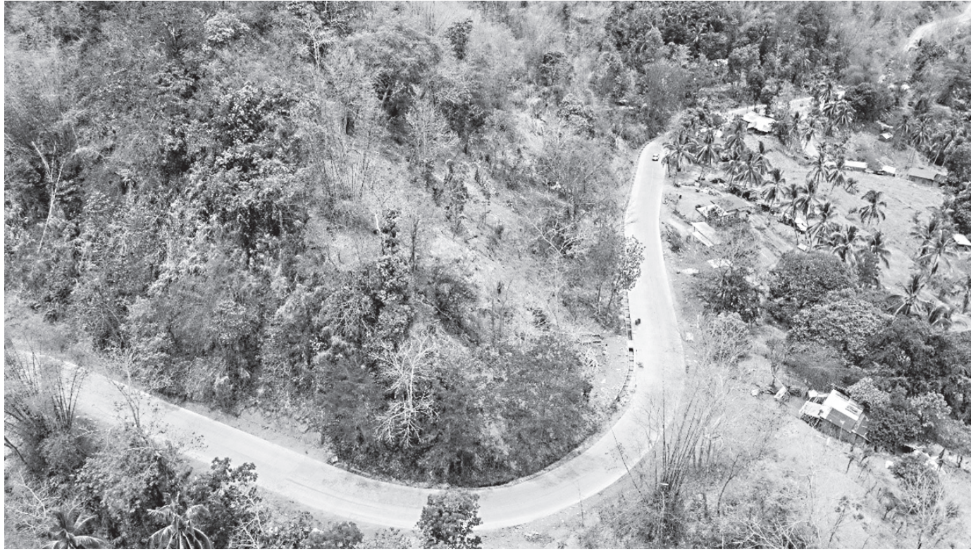
The rehabilitation of the paved roads along junction Bancal-Leon-Antique boundary in the villages of Anonang, Talacuan and Tagsing in Leon, Iloilo has been completed by the Department of Public Works and Highways (DPWH) Iloilo 4th District Engineering Office. (Photo courtesy of DPWH Iloilo 4th DEO)
