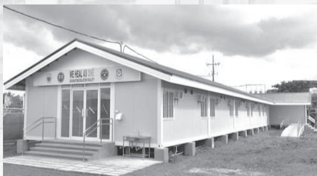
Quarantine / Isolation Facility Brgy. Sooc, Arevalo, Iloilo City
