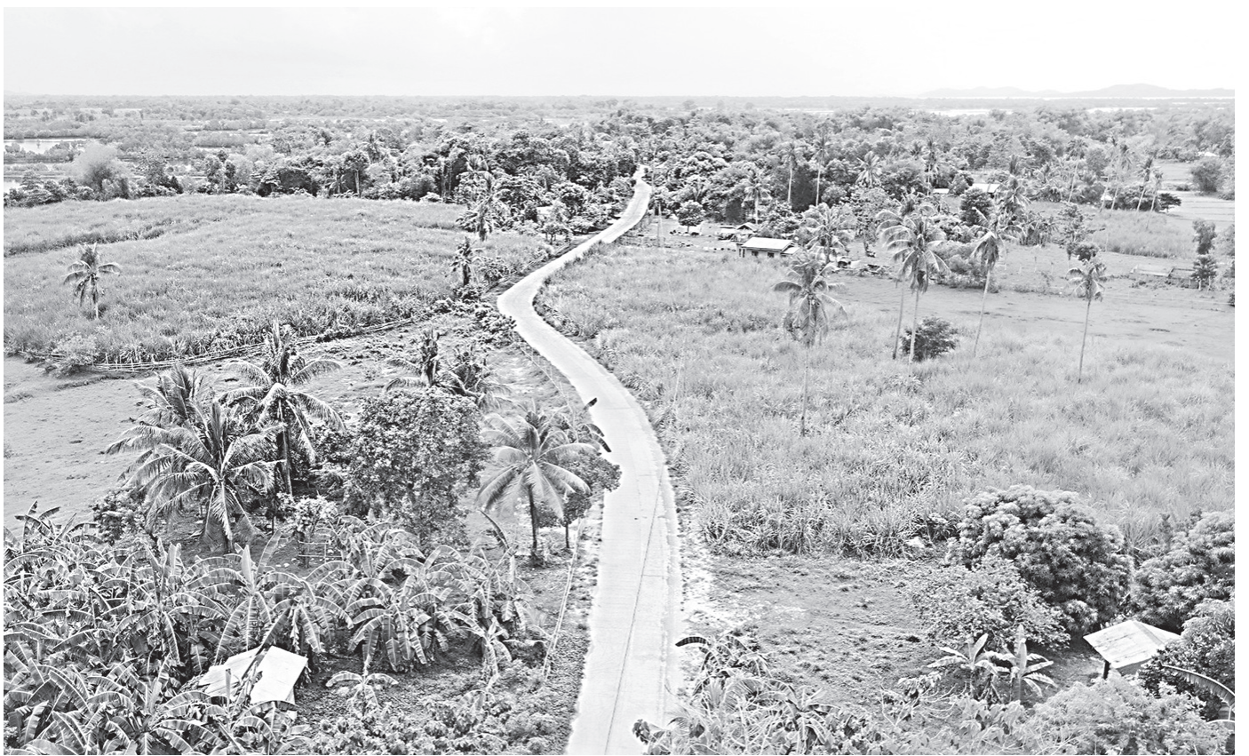
The completed one-kilometer-long farm-to-market road in Barangay Tupaz, Carles, Iloilo aims to enhance local agricultural connectivity. Its construction is through the convergence program of DPWH and the Department of Agriculture. (Photo courtesy of DPWH 6)
