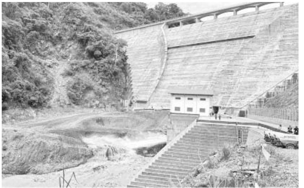
JALOUR DAM. The Jalaur River Multi-Purpose Project Stage II in Calinog, Iloilo, tagged as the largest water reservoir project of the National Irrigation Administration outside Luzon. It is expected to expand NIA's irrigation service by 9,500 hectares, benefitting 7,000 farmers across 17 towns in Iloilo. (PNA file photo)
