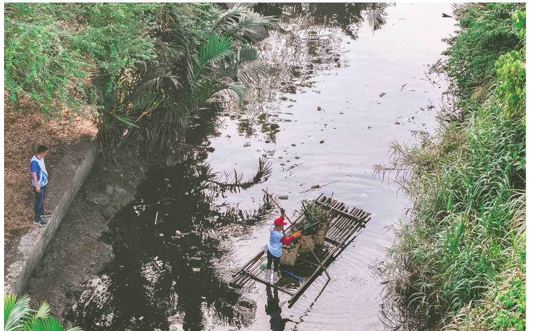
A worker aboard a bamboo raft sifts through a creek in Barangay Ticud, La Paz to remove garbage blocking the water's flow. The Department of Public Works and Highways (DPWH), Department of Labor and Employment (DOLE), and the Iloilo City Government recently launched Oplan Kontra Baha to clear waterways ahead of the rainy season. (DPWH-6 photo)
